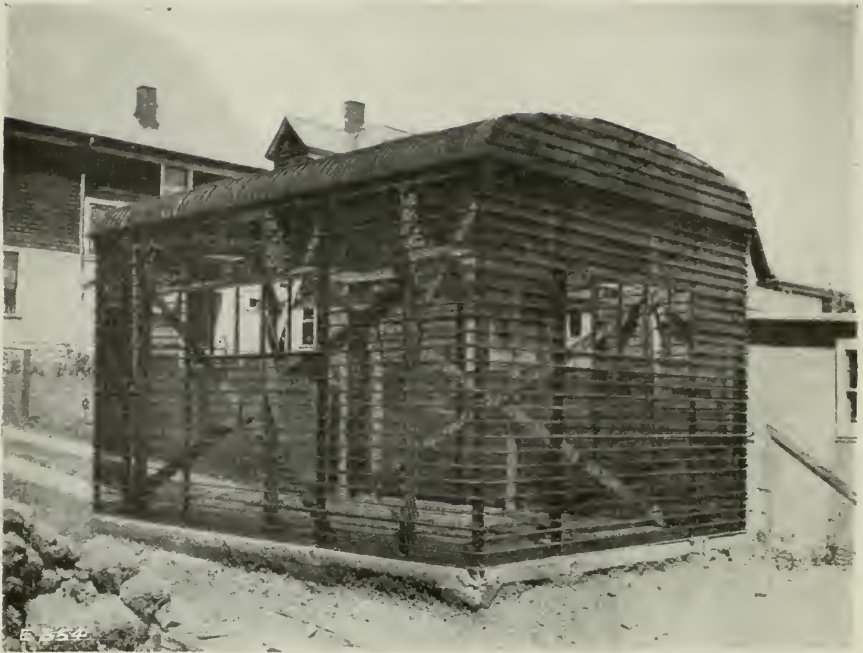
FIG. 53.—METAL LATHING FRAMEWORK FOR SMALL GARAGE.
